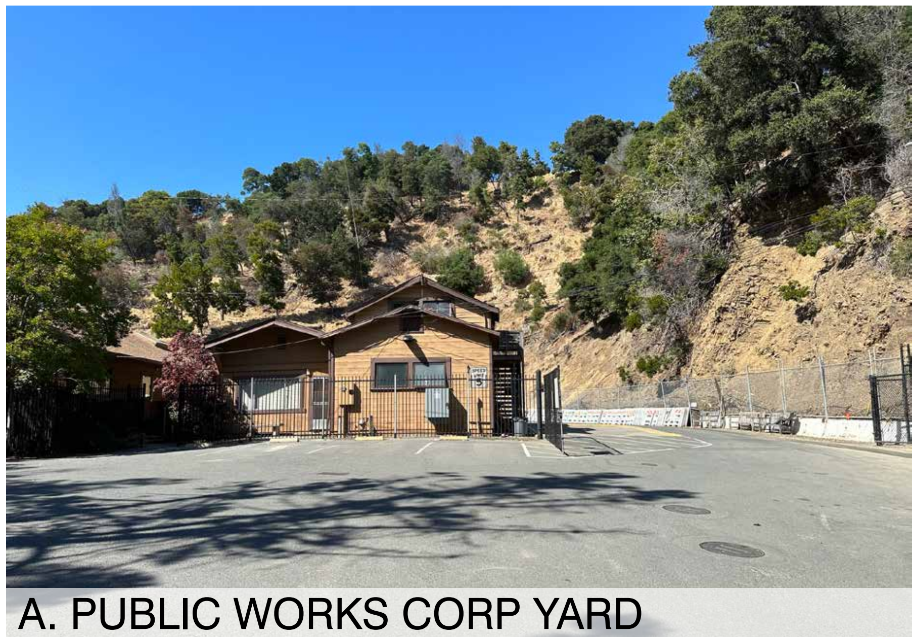
A. PUBLIC WORKS CORP YARD
