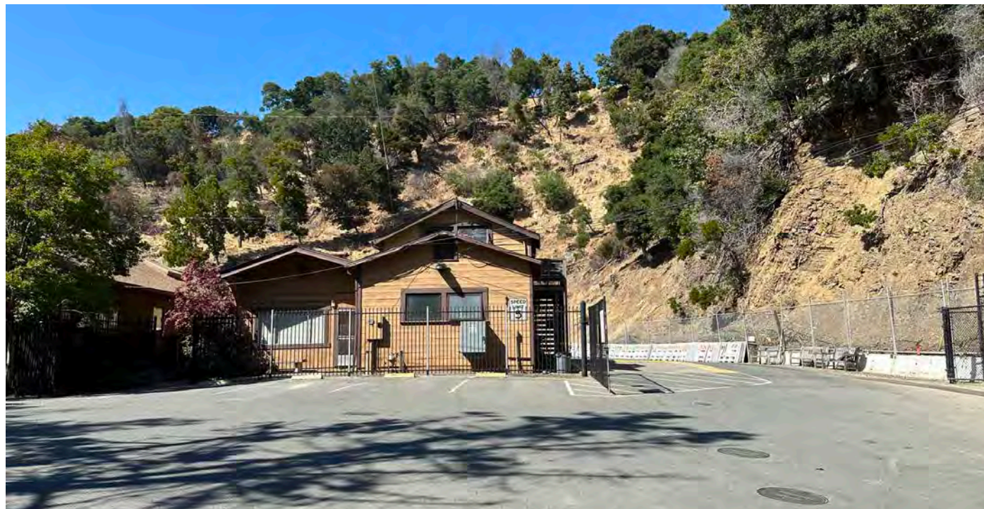
EXISTING CORP YARD OFFICE
