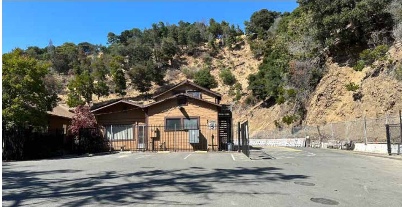
EXISTING CORP YARD OFFICE
