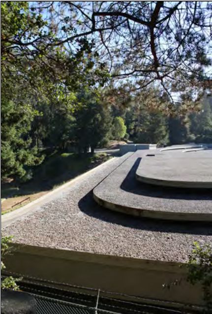
EBMUD's Piedmont Reservoir
